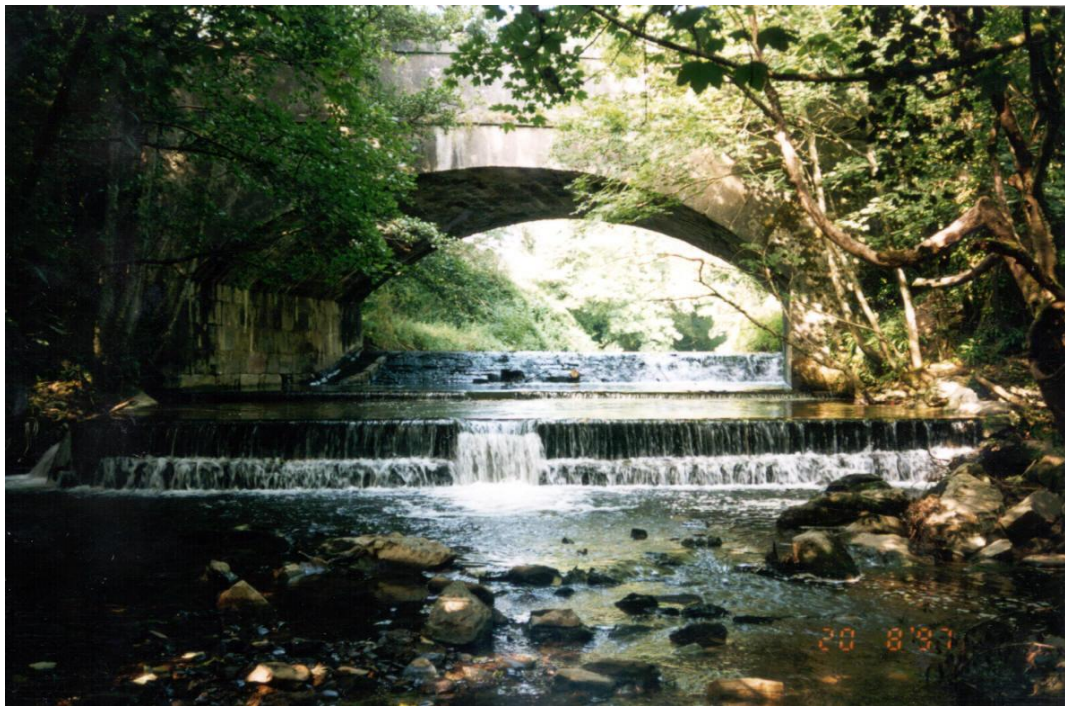
Photo 1. Yealm Bridge and weirs
